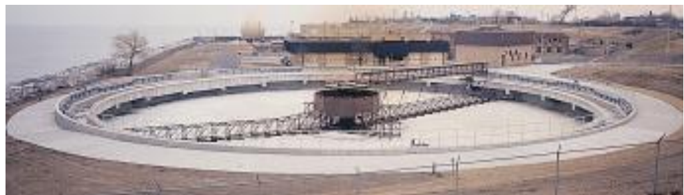
Storm water clarifier installation with walk through truss bridge
