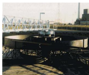
Half Bridge truss formed rake Center Drive Clarifier
